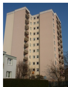
Figure 2. Building with a cable-driven elevator
